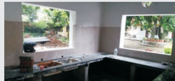
▼ Construction of the Kitchen building in full-swing
